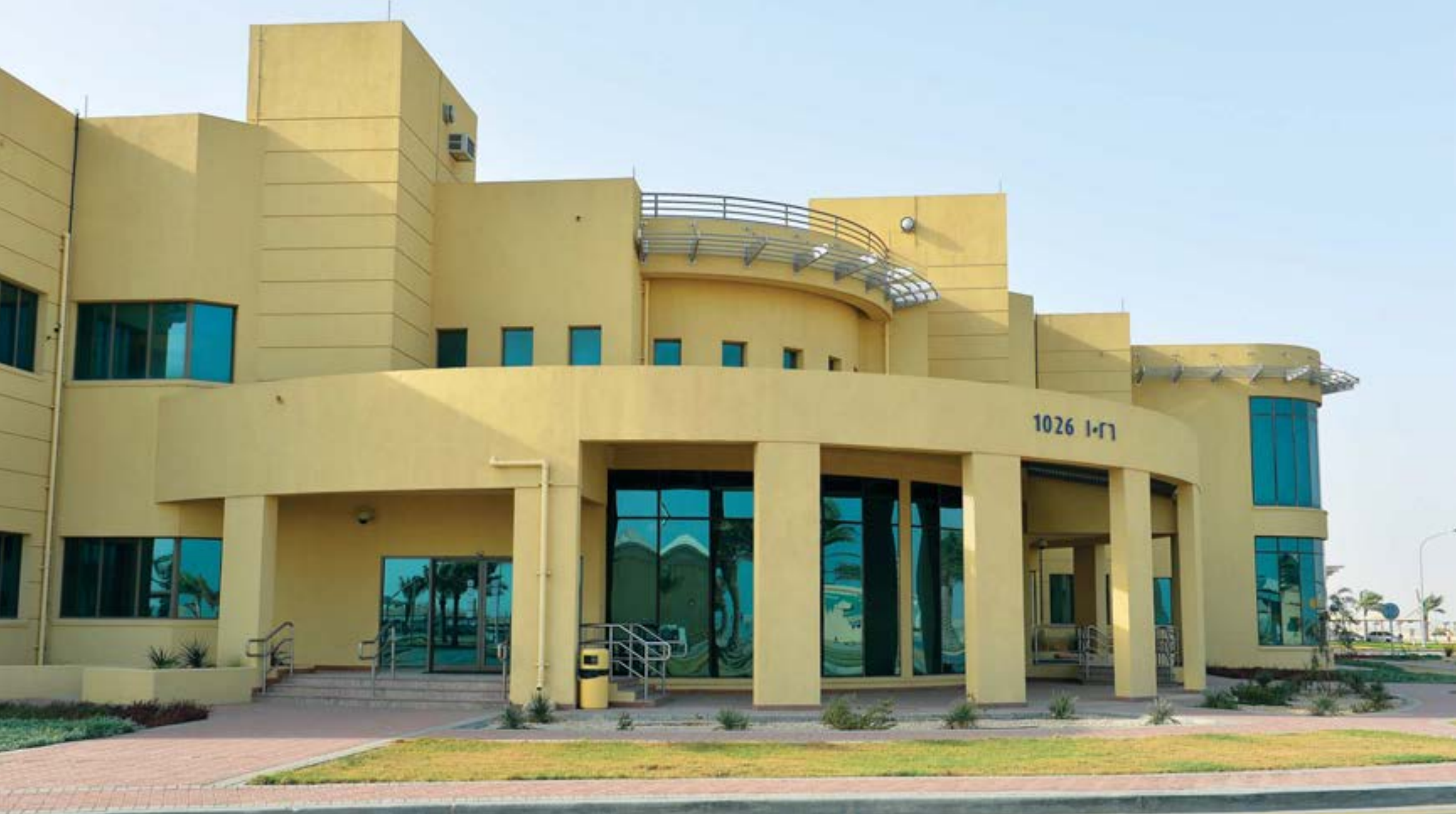
Manifa Producing Department Administration building
